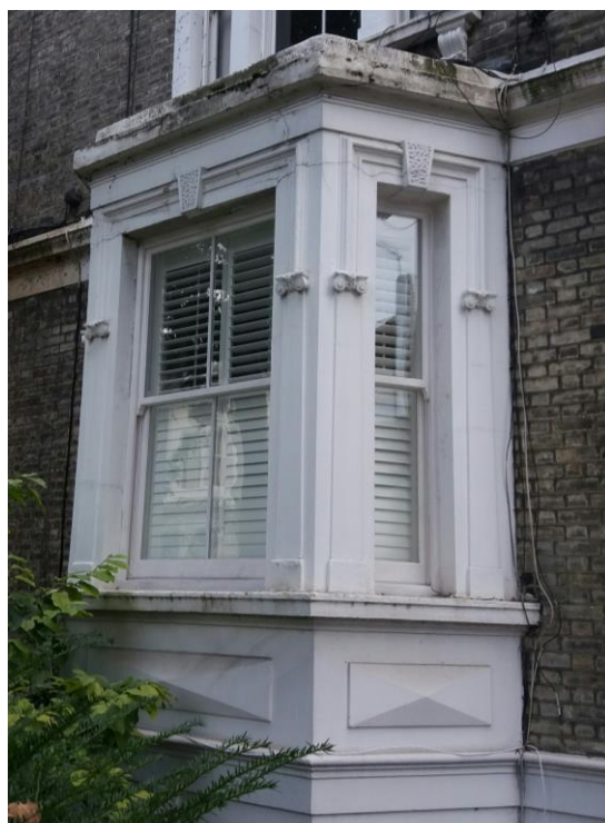
Ornate stucco decoration on the bay of no. 2 Barclay Road.
