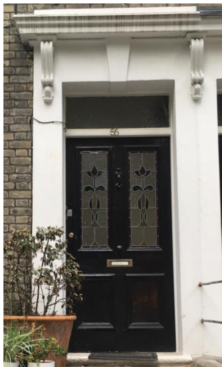
Stained Glass door panels, no. 56 Barclay Road.
