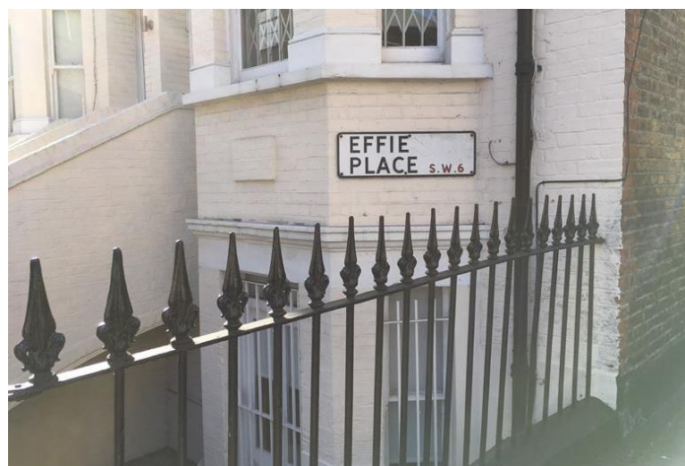
Bridge over lightwell to entrances and old street name plate. Effie Place.
