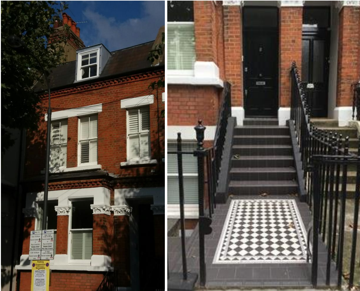
No. 9 Barclay Road with original red brickwork and recently restored black painted railings and sympathetic tiling.
