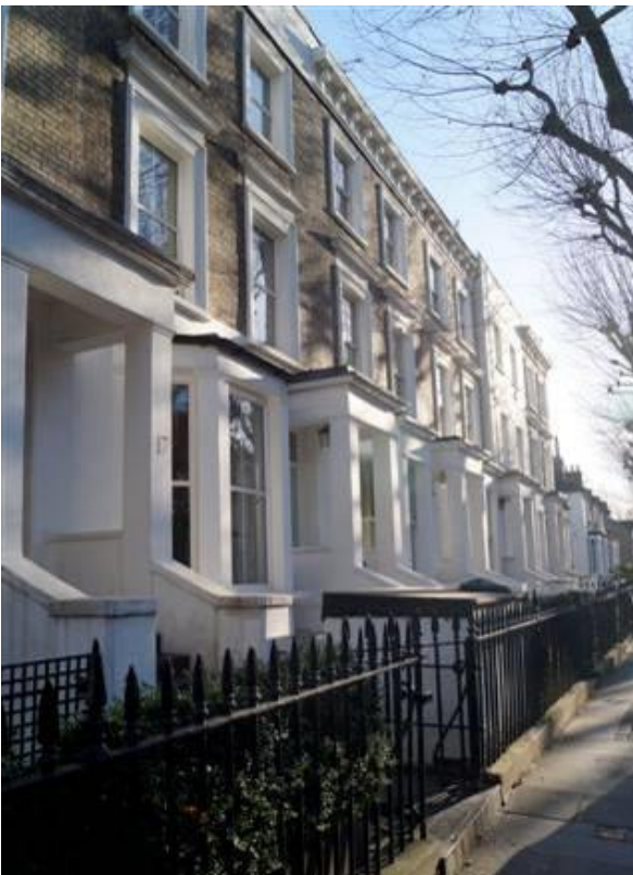
No. 17-25 (odd) Barclay Road, with finial topped railings.
