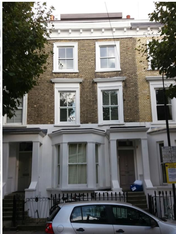
Restored cornice and modern roof extension behind the parapet, no. 21 Barclay Road.
