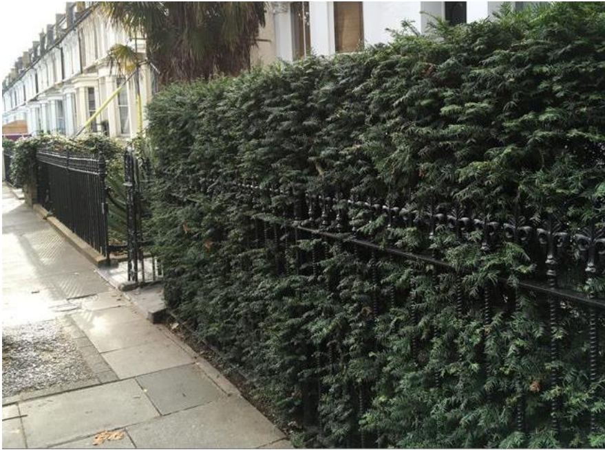
Original iron railings.
