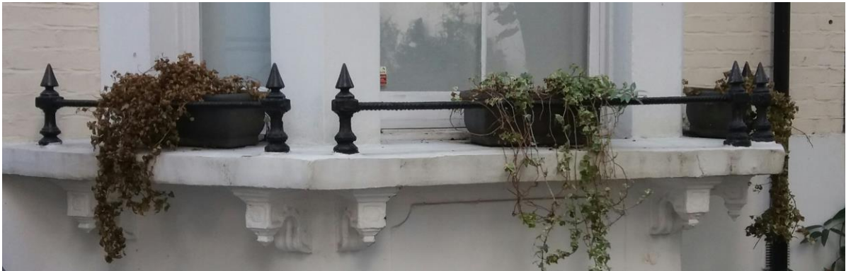
Original wrought iron window sill castings.
