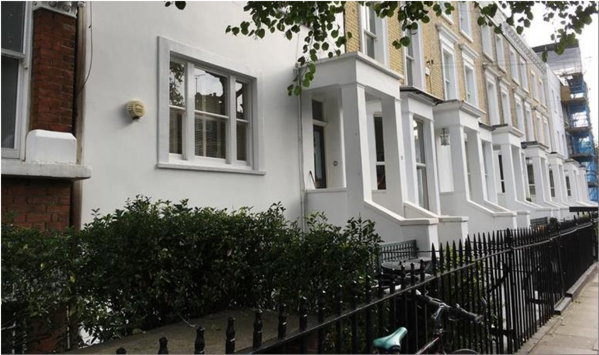
Unfortunate loss of bay and rendered façade, no. 13 Barclay Road.
